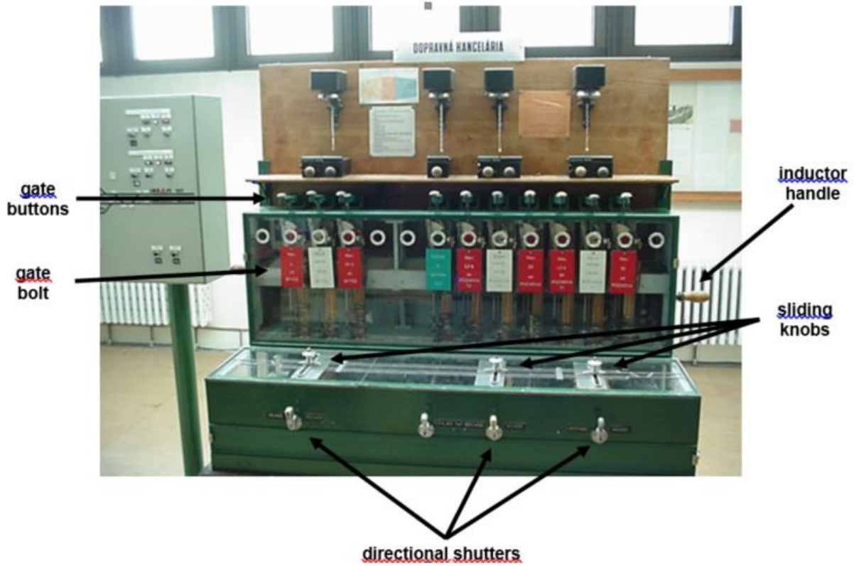
Figure 9 Control elements on the electromechanical safety device (controlling interlocking box)
